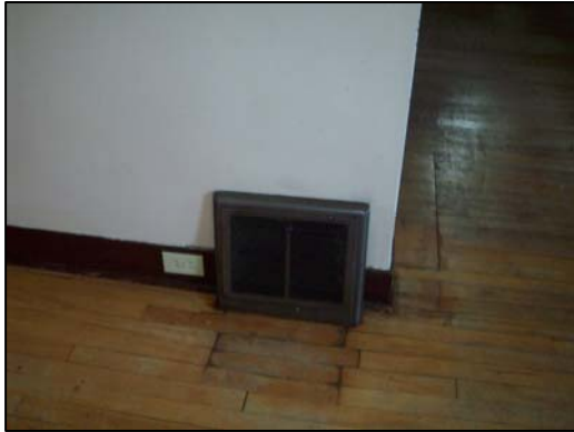
Example of Duct Wrap - Friable Register Boots/Runs Throughout
