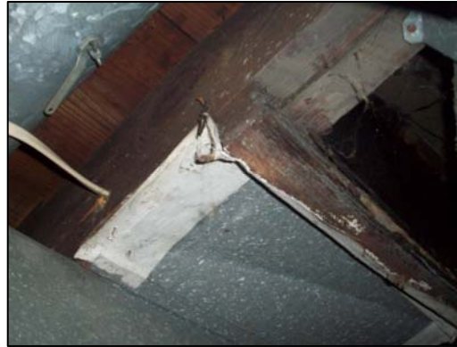
Example of Duct Wrap Tape - Friable Basement
